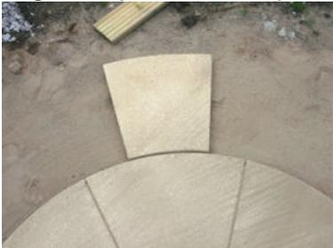
then check with a spirit level to make sure that the first slab ring is level or, in the case of large patios, has a slight fall to one side to shed rain water.
